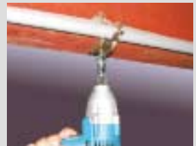
Installing piping or wiring supports
