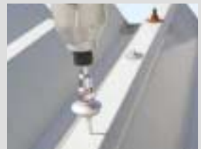
A ring nut setter is the best choice for securely fastening drill screws or flanged hexagon head screws with in high places as when anchoring angled plates in the middle.
