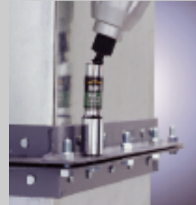
Tightening of duct coupling
