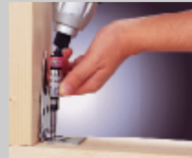
Installing tension and angle brackets
