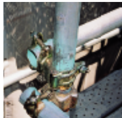
Tightening of step clamp
