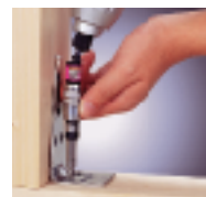
Installing tension and angle brackets
