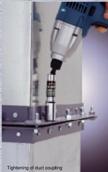
Tightening of duct coupling
